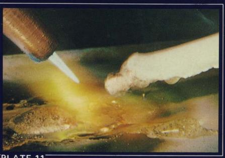
PLATE 11 The brazing rod is dipped into the leading edge of the braze pool.
