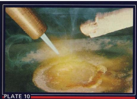
The base metal is heated and the brazing rod is touched to it to determine if the brazing temperature has been reached.
